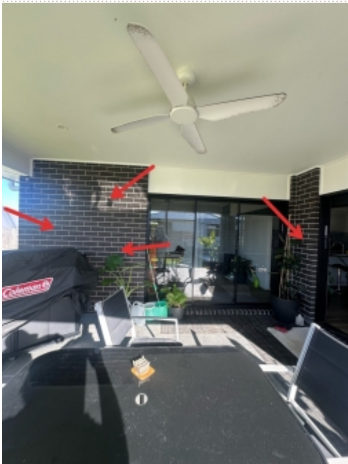
Photo(s) of Defect
